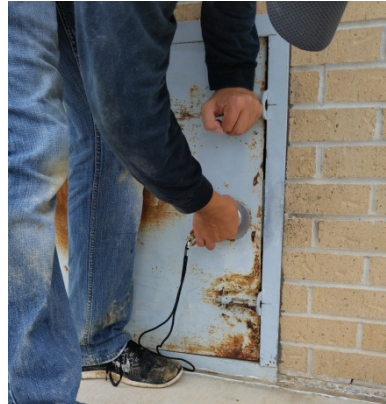
Door bent & could not be opened
