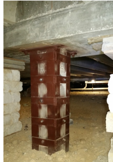
Column jacketed with steel retrofit and supported on either side by stacked masonry
