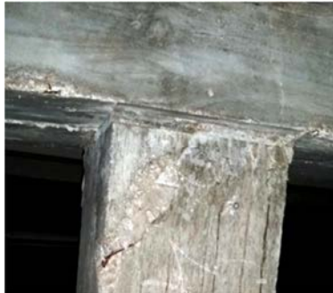
Diagonal crack at top of column, Minor beam and column spalling/honeycombing
