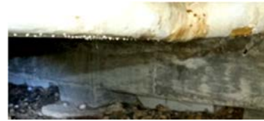
Condensation on pipe
