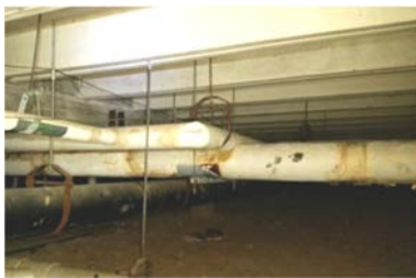
Pipe insulation in poor condition
