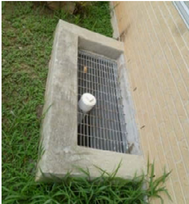
Areaway with grate welded down
