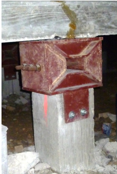
Column retrofit steel "box" Epoxy injected crack in beam above column
