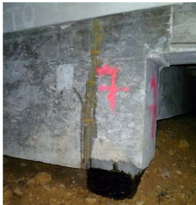
Beam with large crack that was epoxy injected
