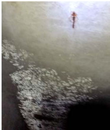
Exposed reinforcement under precast slab. Condensation under slab.
