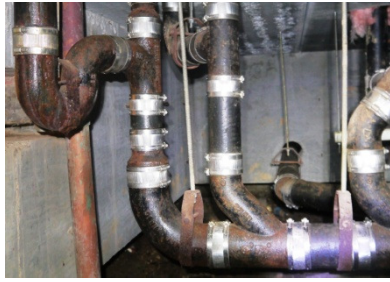
Minor rusting in cast iron pipe and rusted hangers
