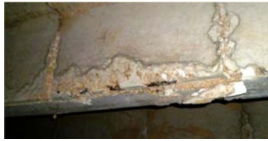
Honeycombing/spalling/corroded reinforcement at pan joist
