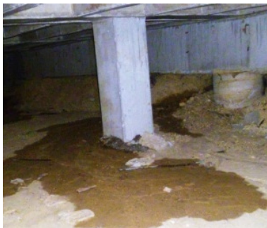
Water infiltration at building perimeter
