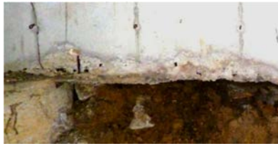
Honeycombing/spalling/rusted reinforcement at bottom of perimeter beam
