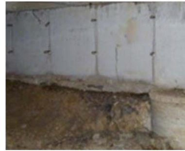
Soil in contact with bottom of perimeter beam
