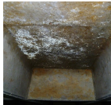
Condensation on underside of slab indicates poor ventilation
