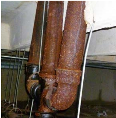
Corrosion in cast iron pipes
