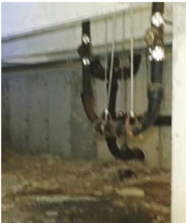
Leaking cast iron pipe
