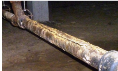
Cracked cast iron pipe
