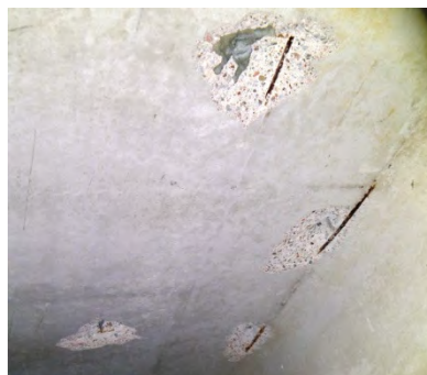
Spalleg, expgseg/cgrrg eg reigf area ig g precast geck g
