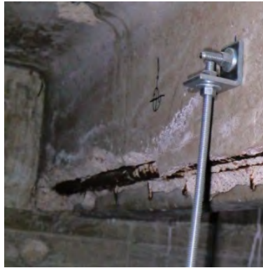
Sig ificagt spallig ag expgseg/cgrrg eg g reigfgrcemegt ig precast pag jgist webs g
