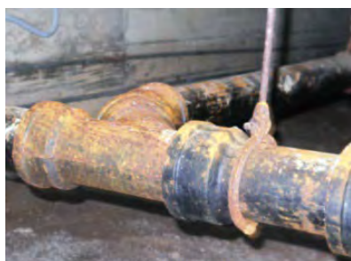
Rusted cast iron pipes and pipe hangers
