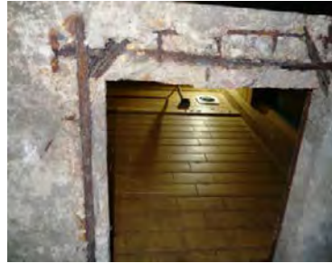
Exposed/corroded reinforcement at C Wing floor hatch
