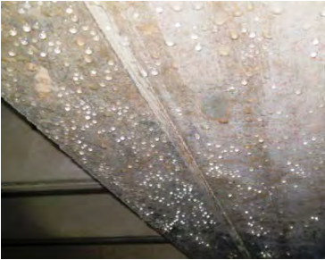
Condensation under beam indicates poor ventilation
