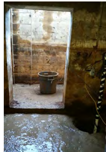
Mud at bottom of vault under gym and sump pit observed November 14, 2016 (after standing water removed).
