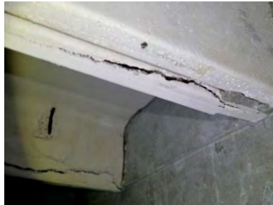
Longitudinal cracks along bottoms of precast channel legs
