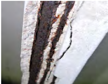
Advanced corrosion & scaling on channel leg longitudinal reinforcing
