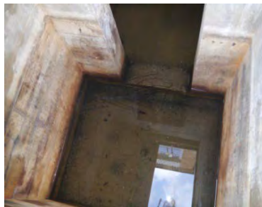
Standing water in vault access on November 2, 2016.
