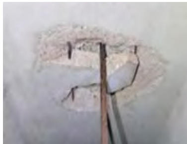
Slab spalling at pipe hanger connection
