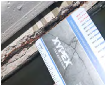
Channel leg exposed longitudinal bar has less than 1/2in of clear cover to outside face of concrete
