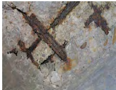
Slab spalling & corroded rebar
