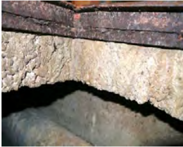
Slab honeycombing and corroded steel frame at C Wing floor hatch
