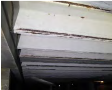
Longitudinal spalling & corroded/scaling reinforcement along bottoms of precast channel legs
