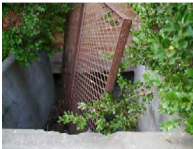
Kitchen crawl space areaway opening too small to access
