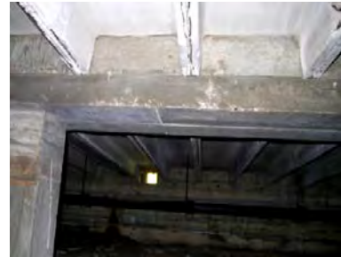
Longitudinal spalling & corroded/scaling reinforcement along bottoms of precast channel legs
