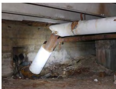
Degraded pipe insulation
