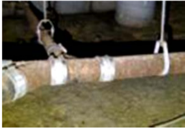
Rusted cast iron pipes
