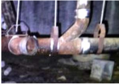
Broken pipe and rusted hangers
