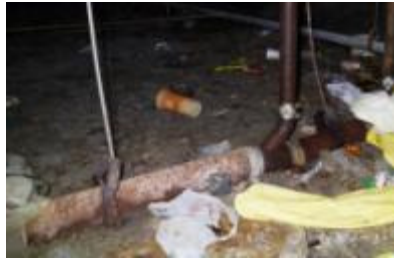
Pipe on the ground, failed hangers
