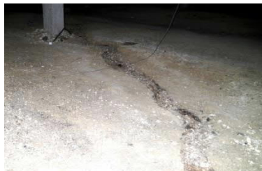
Water trails in soil indicate running surface water in crawl space
