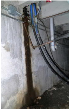
Leaking pipe
