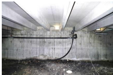
Damp soil adjacent to perimeter beams
