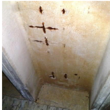
Exposed pan joist flange reinforcement
