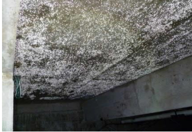
Condensation on underside of floor structure
