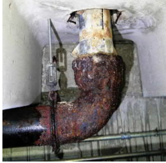
Corroded pipes
