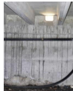
Inadequate ventilation in perimeter beams
