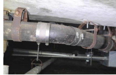
Corroded hangers
