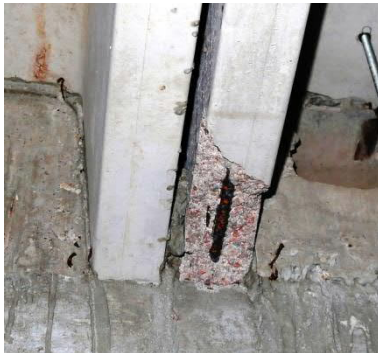
Pan joist web spalling at beam support
