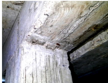
Minor beam spalling & corroded reinforcement
