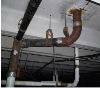
Corroded pipes
