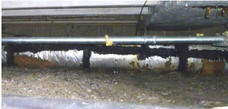
Duct is torn & losing insulation
